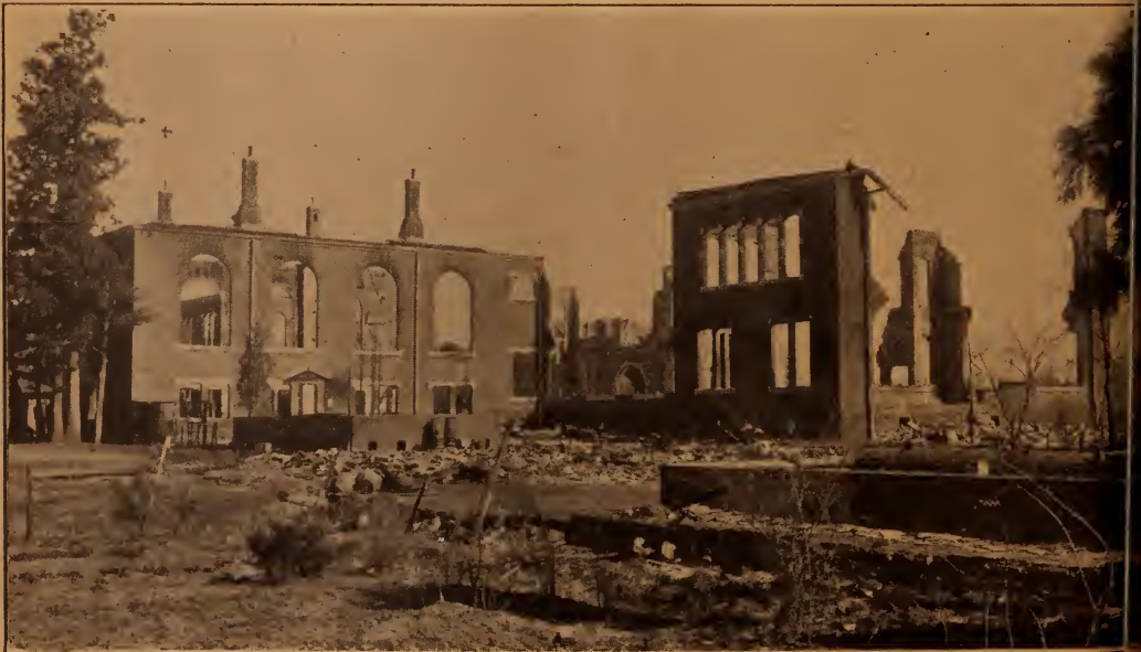
RUINS OF NORTH JAPAN COLLEGE BUILDING.
